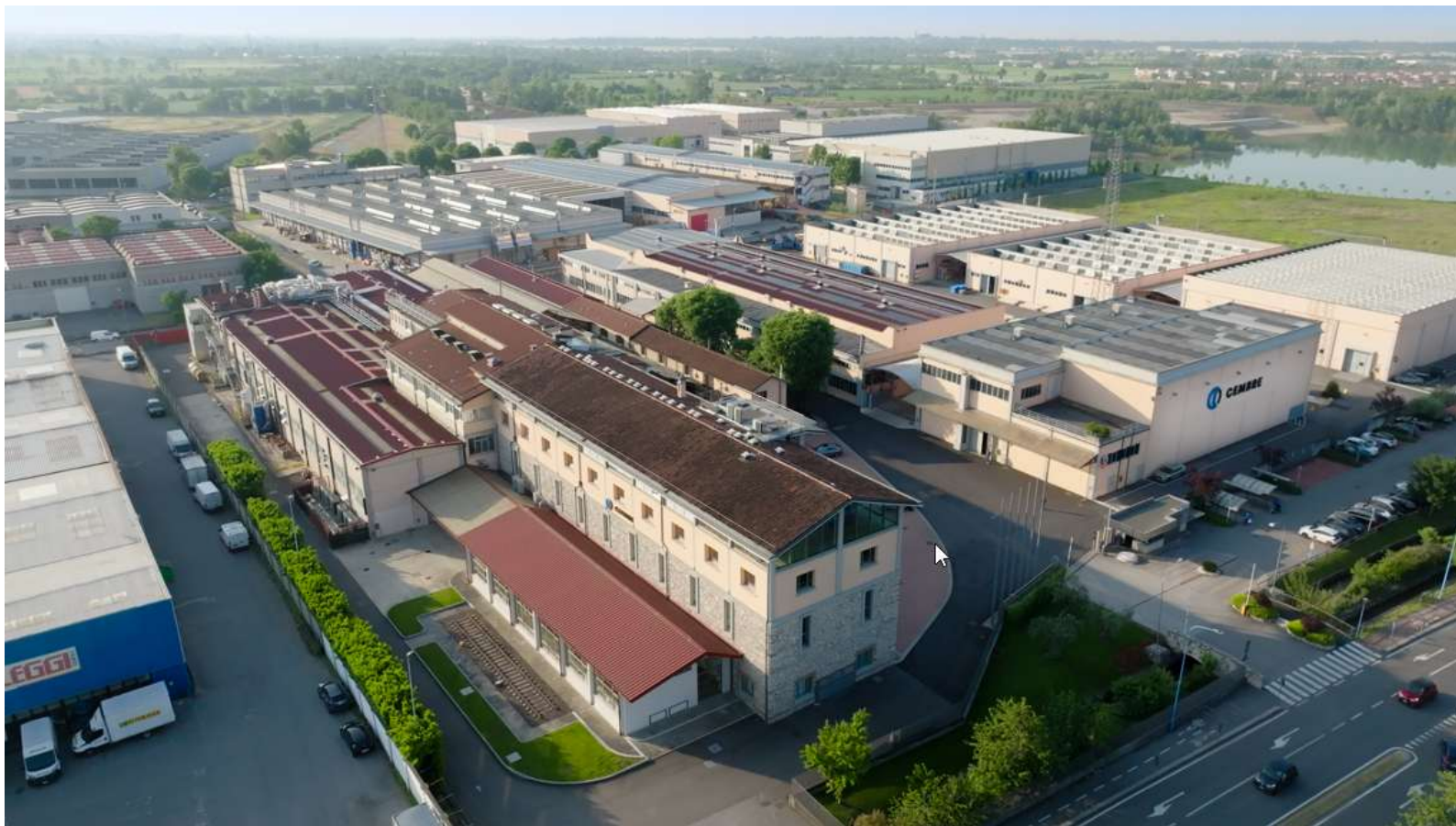
CEMBRE S.p.A. – Headquarter in Brescia (Italy)
