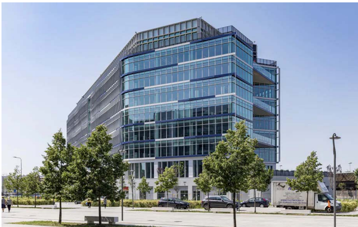
SAIPEM HEAD OFFICE, Spark 1
