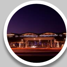
Riyadh Metro Line 3 Saudi Arabia
