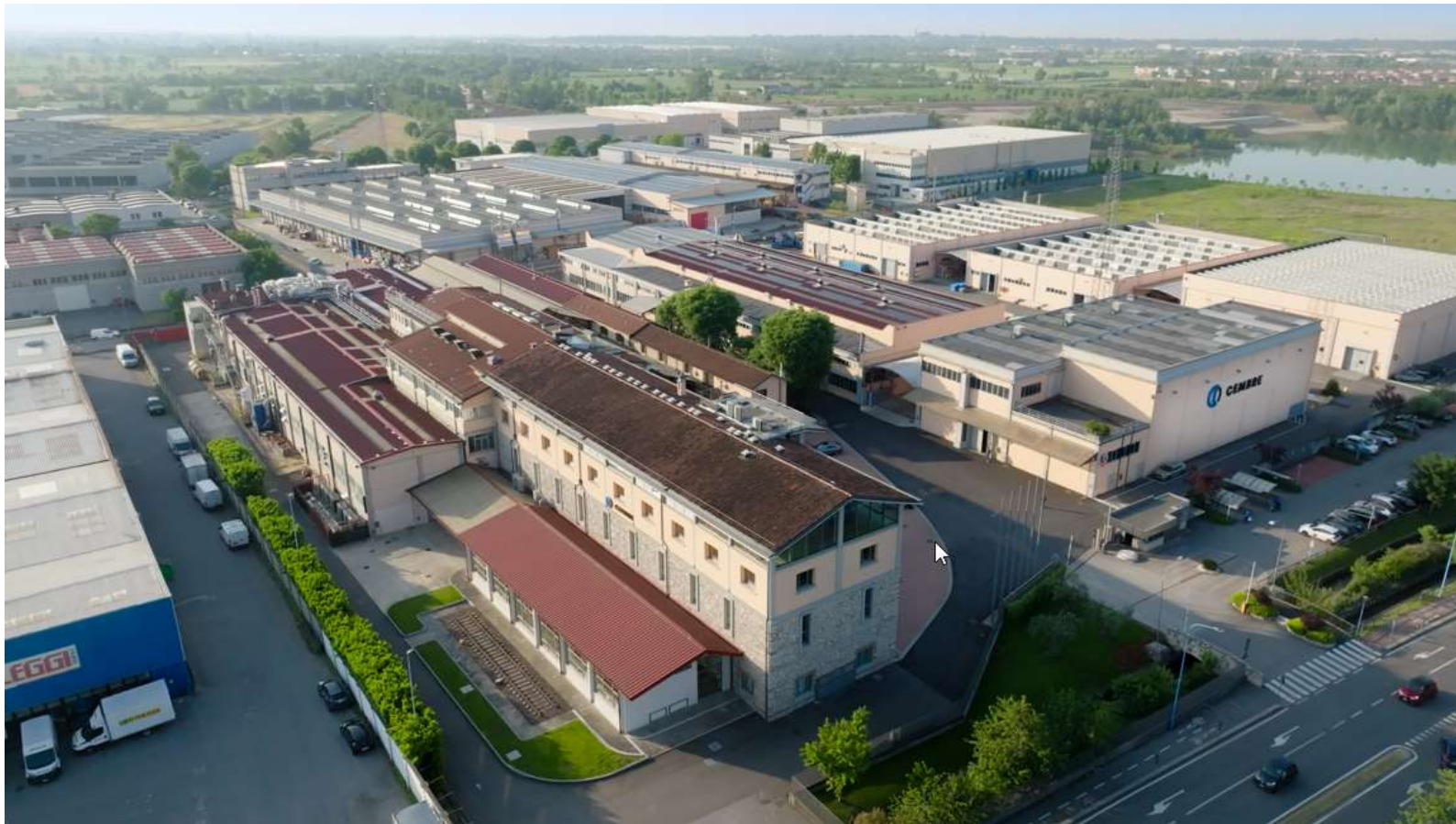
CEMBRE S.p.A. – Headquarter in Brescia (Italy)
