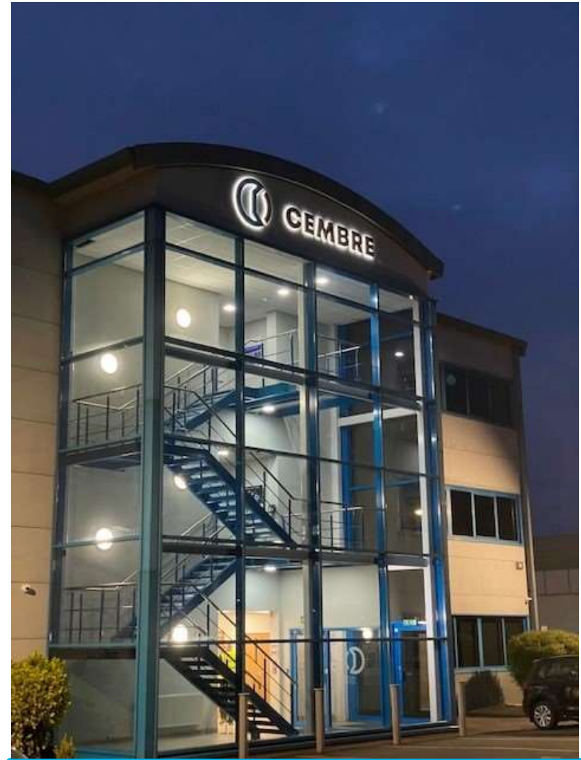
CEMBRE Ltd. – Factory in Curdworth Birmingham (UK)
